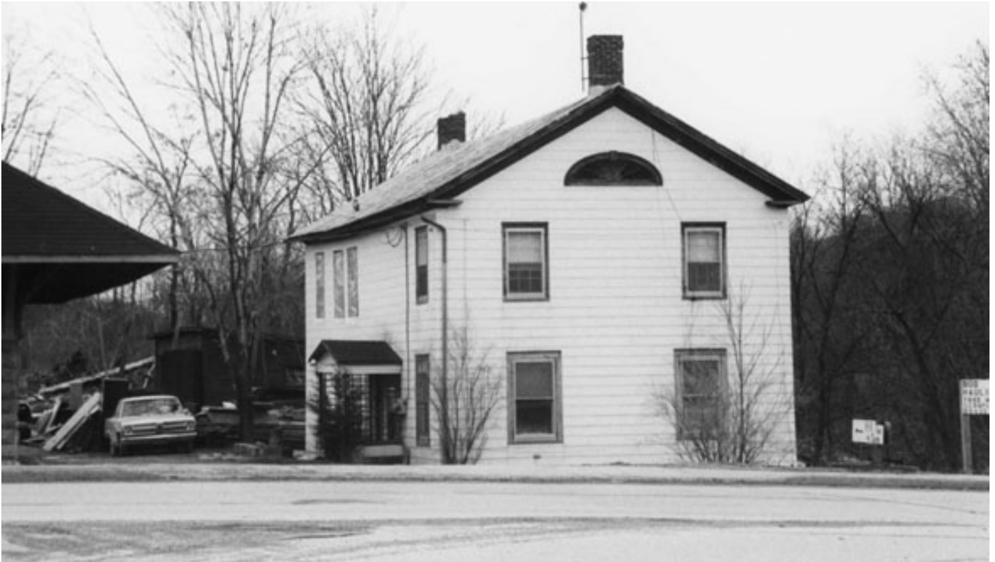
Fig.4: Photograph of Mill Office from the South, January 1981. Neil G. Larson, "National Register of Historic Places nomination, Wild's Mill Complex" (New York State Office of Parks, Recreation and Historic Preservation; December 1981).
