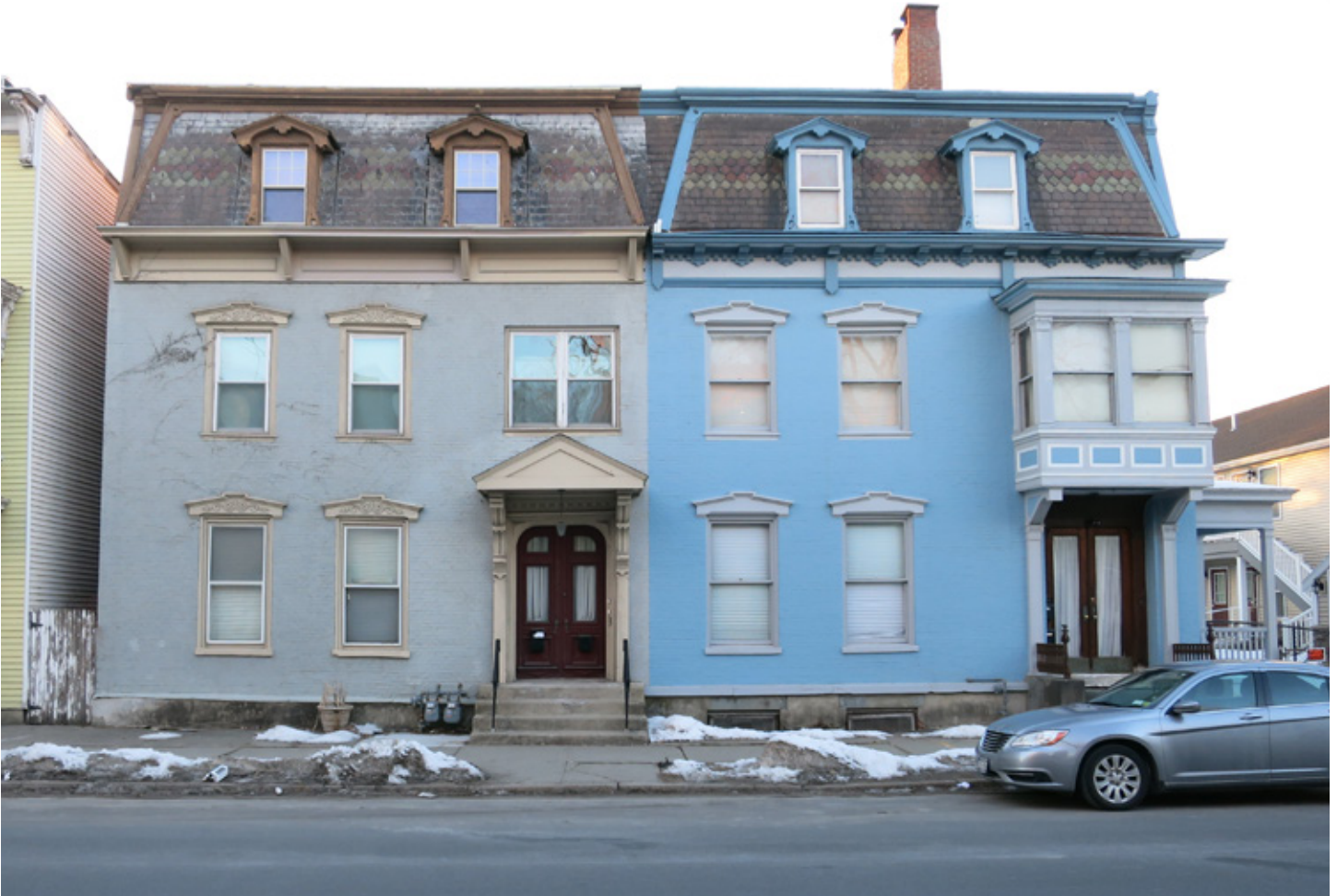
Fig.5: Henry-Alvord-Burton Houses, ca. 1790 & ca. 1879, 551-553 Second Ave. These two townhouse-like residences disguise an older five-bay, center-hall residence built ca. 1790 with a gambrel roof that was later modified into a mansard to accommodate the addition of a sixth bay. Photo by SHPO staff, 2022.
