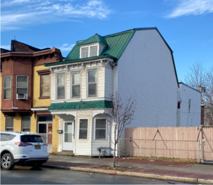
Fig.3: Fitch Skinner House, ca. 1800, 513 ½ Second Ave. This house is an example of a wood clapboard sheathed Dutch gambrel-roof hybrid. It was the home and workshop of Fitch Skinner (1777-1844), a well-respected master cabinetmaker from East Windsor, CT, in the early part of the nineteenth century.
