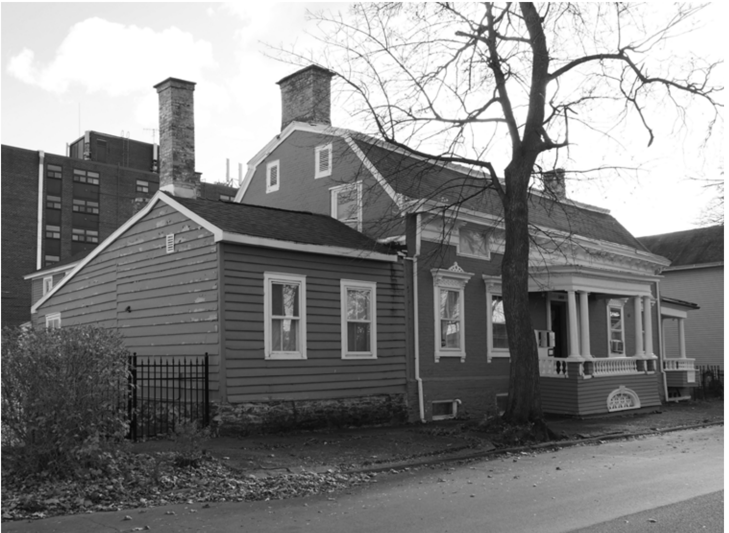
Fig 2: Unknown merchant's house, ca. 1775, 580 First Ave. This is the only story-and-a-half brick house with a gambrel roof found (so far) in Lansingburgh.
