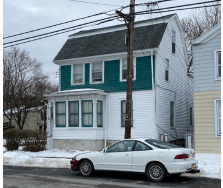
Fig.4: James Boggs Jr. House, ca. 1790, 499 Sixth Ave. The facade of this early wood clapboard house was later updated to reflect contemporary architectural trends, as is the case with most of the early examples in the district.
