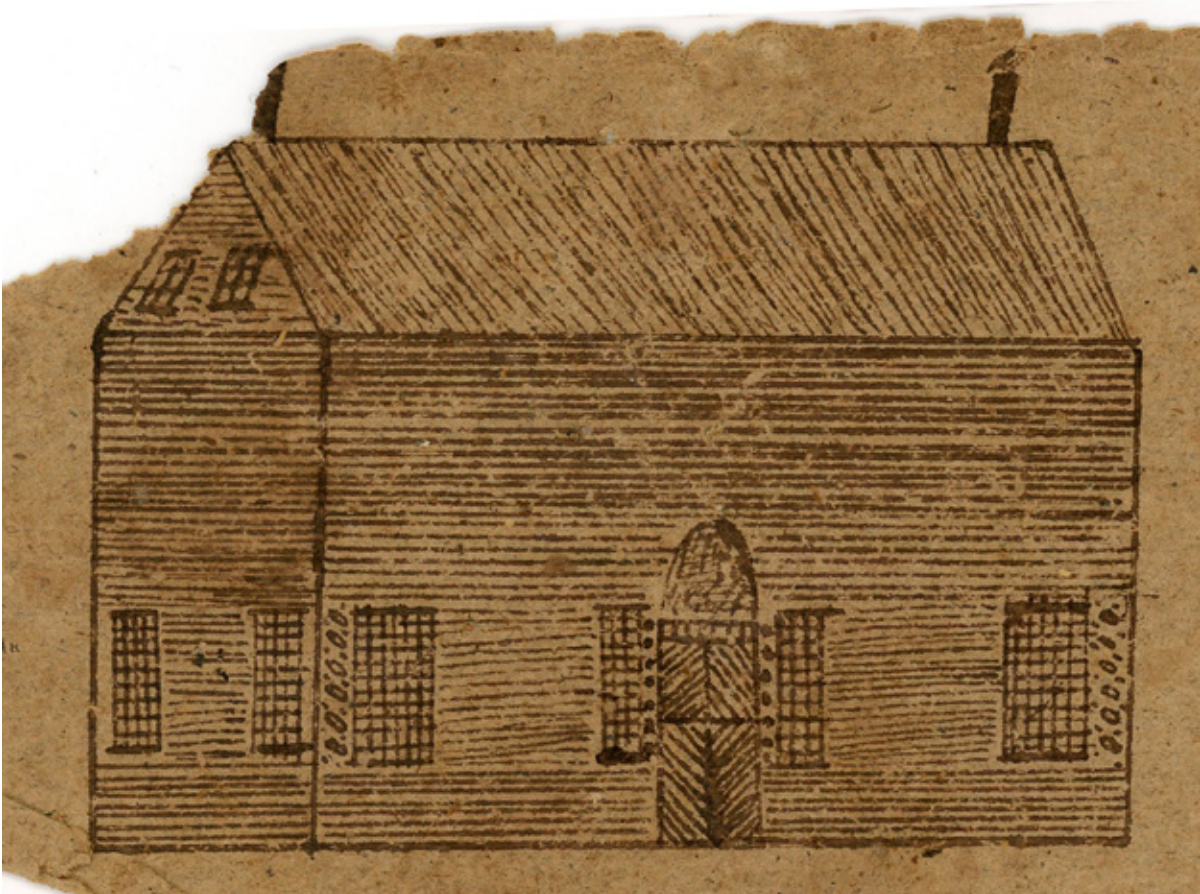
An early 19th century drawing found in the family papers of William Becker (1774-1838) and Catherine Margaret Blass Becker (1781-1824) of Germantown, believed to depict their house (Collection of Rachel Clothier). Typical of rural wood framed dwellings constructed in the Hudson and Mohawk valleys in the 1790-1825 period, structures such as this were commonly framed using a series of parallel H-bents, following New World Dutch building traditions. A contemporary example survives on Wood Lane in Salem, Washington County. (See below)
