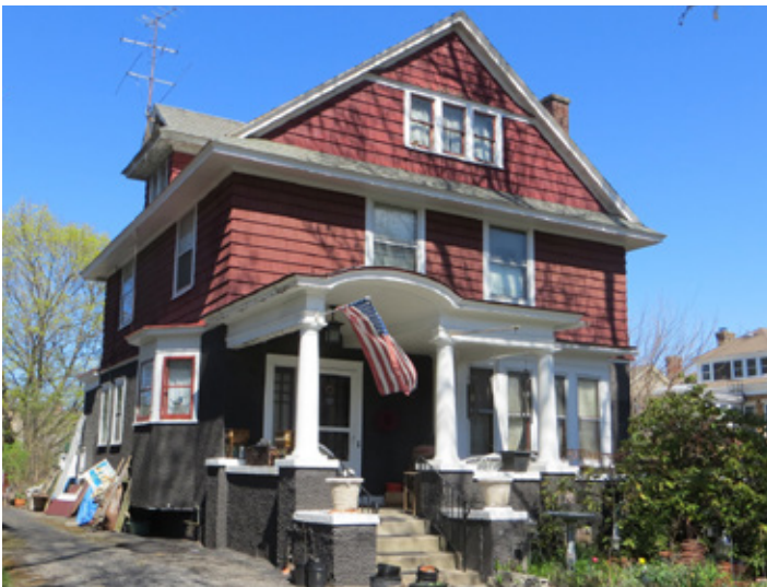
Fig. 2: Lindsay-Holtzmann House, 2 Morris Ave., 1912, from south.
