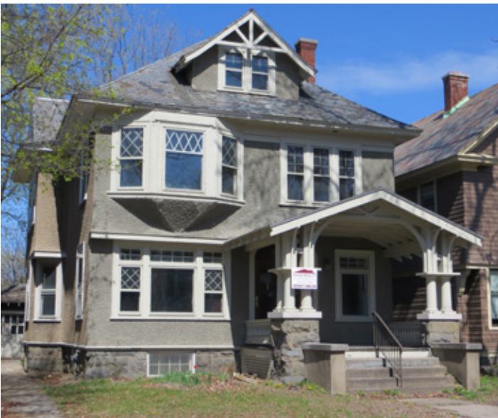
Fig. 10: Veeder-Swick House, 12 Morris Ave., 1913, from south.
