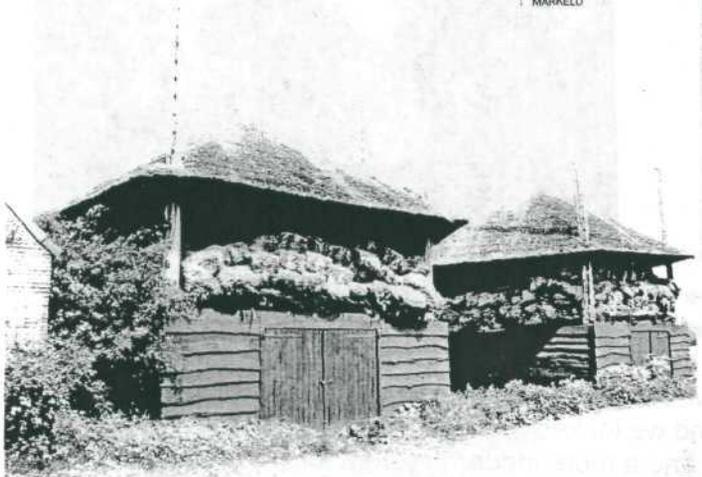
Two 4-Pole Barracks (*steltenbergen*) with raised floor and enclosure along the Linge River
