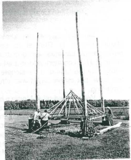
pair above the other. I had surmised for the New World rafter system the four major rafters joining to a center block. This should be rethought. The Dutch system allows for flexibility.
