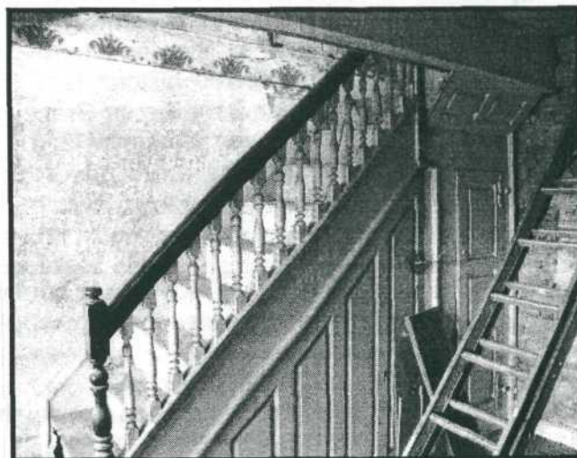
1766 Newel-Post, Hand-Rail and Stairs Conyn/Van Rensselaer House Claverack, Dutchess County, NY (NY/Col/Cla/06)
