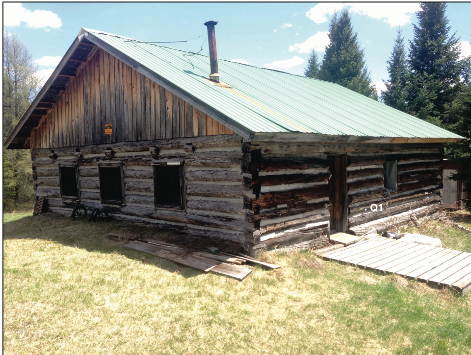
Figure 8. Sample location (Q) on the west side of the cabin.
